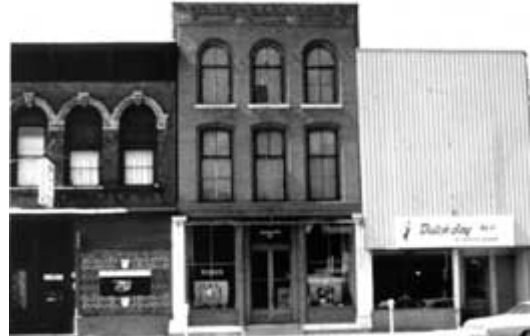
This photograph shows the impact of preserving historic storefronts. The one on the right has been totally obscured by a "modern" front added in the 1950s. Photo: NPS files.
