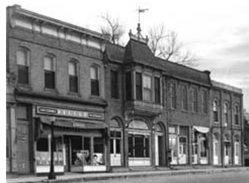
By evaluating the components of a storefront as well as their existing condition, a successful rehabilitation is more likely. Photo: HABS collection, NPS.
