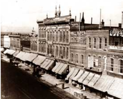
Try to locate old photographs or prints to determine what alterations have been made to the storefront and when they were undertaken. Awnings were common elements of storefronts at the turn of the century. Photo: NPS files
