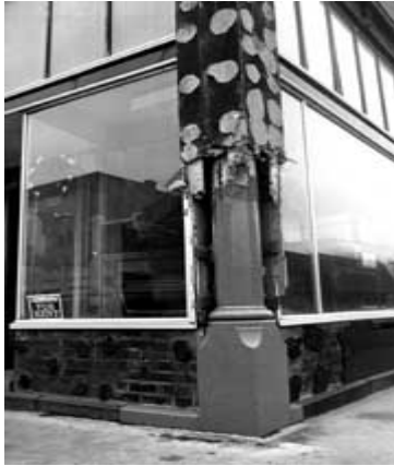
Storefronts of the 1940s, 50s, and 60s were frequently installed by attaching studs or a metal grid over an early front and applying new covering materials. Photo: Bob Dunn
